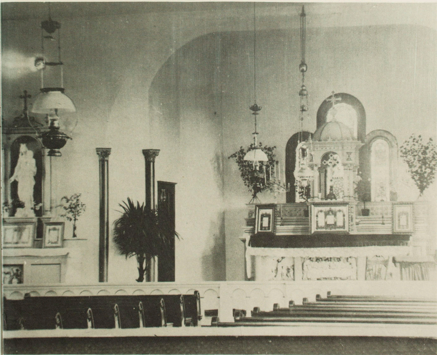
Tiffany light fixtures, rare statues and handmade pine window frames decorated the interior of St. Mary's Catholic Church. The inside walls are of galvanized tin hammered into Florentine design.
