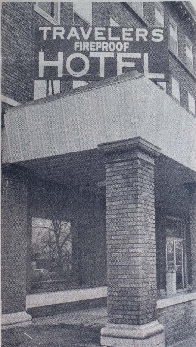
SIGN SLIP-UP -The Traveler's sign remains intact after firemen were able to contain the blaze in the basement.
