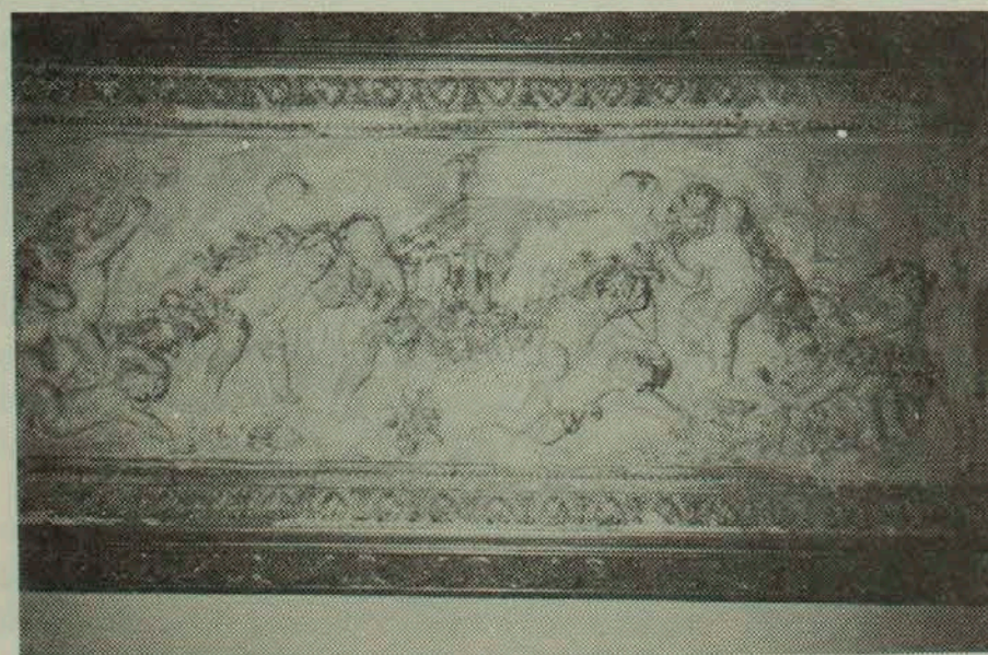
This beautiful fresco is from inside the theatre. It is made of plaster and horsehair; the horsehair was used as a reinforcement to the plaster. (Photo courtesy of Burt Beard)
