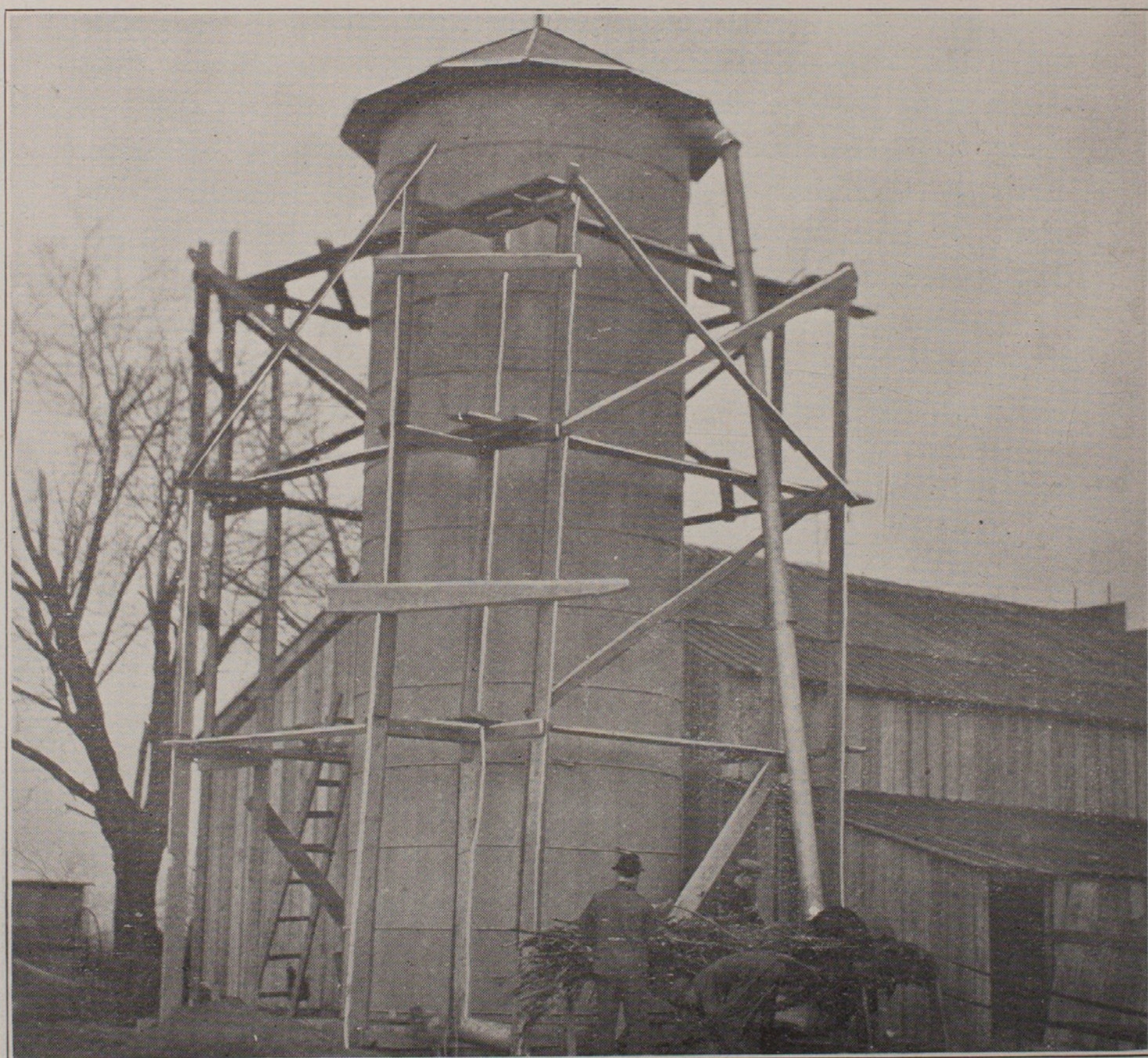
SILO CONSTRUCTED AND FILLED BY STUDENTS OF AGRICULTURE AT SCHOOL FARM.
