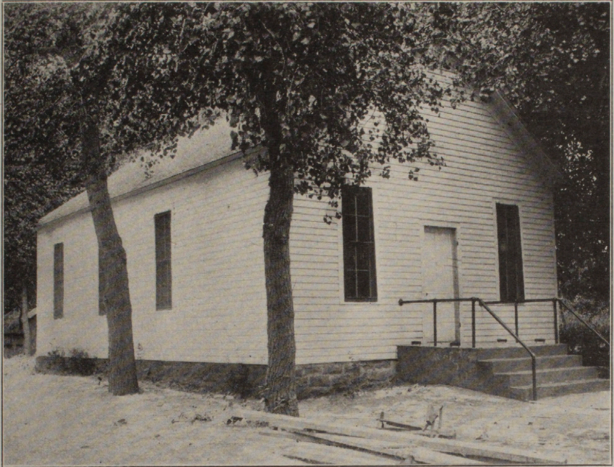
ONE OF THE SIX ORIGINAL SCHOOLHOUSES AT CACHE LA POUFRE SCHOOL
