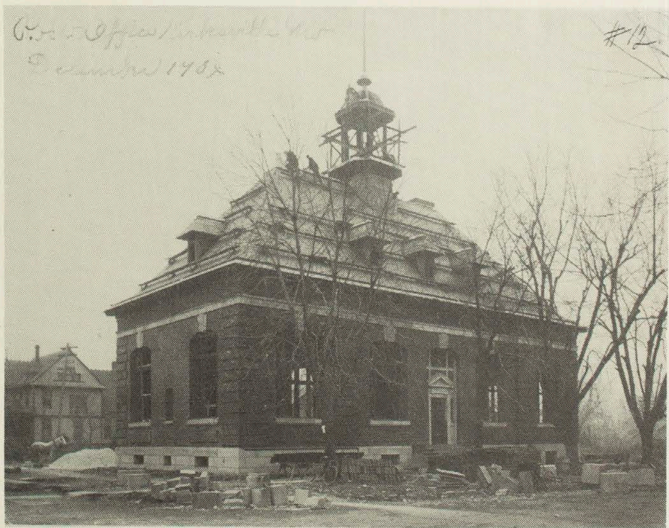
In the top photo, four gentlemen posed at the back of the Post Office in October 1904. The bottom photo is dated December of that year, showing workers putting on the finishing touches to the roof and cupola.
