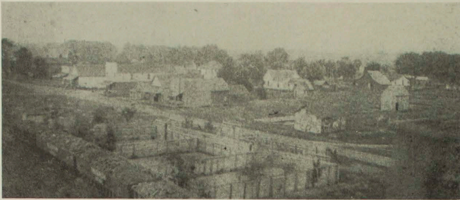
This picture, taken from the coal chute looking north, shows Millard in the early 1900s. (Note the coal trains, with the stockyards and businesses located near the railroad.) Photo courtesy of Jolene Cody.
