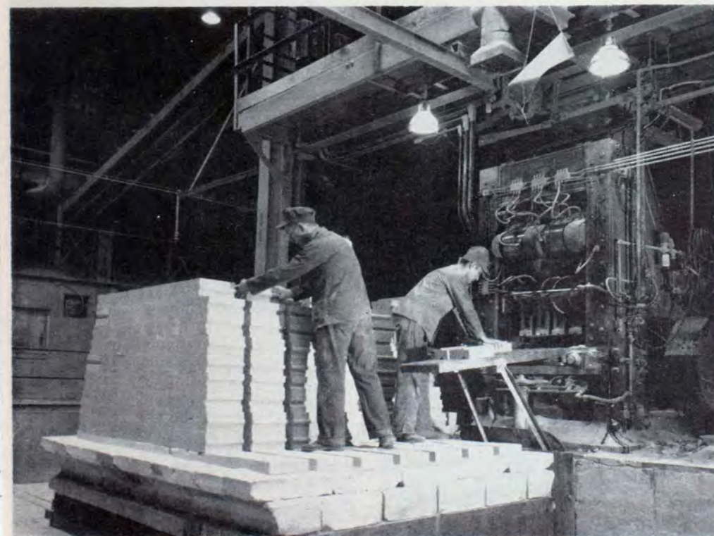
SETTING POWER PRESSED BRICK ON TUNNEL KILN CAR FOR FIRING
