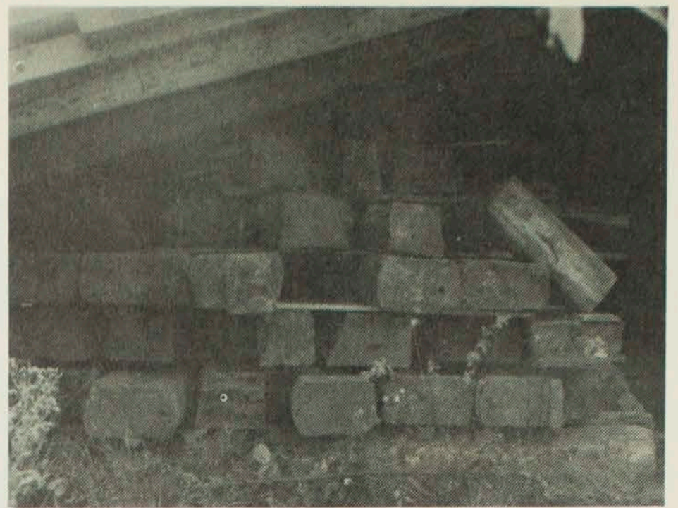
The logs from the house are stacked in sections and numbered to aid in reconstructing the home.
