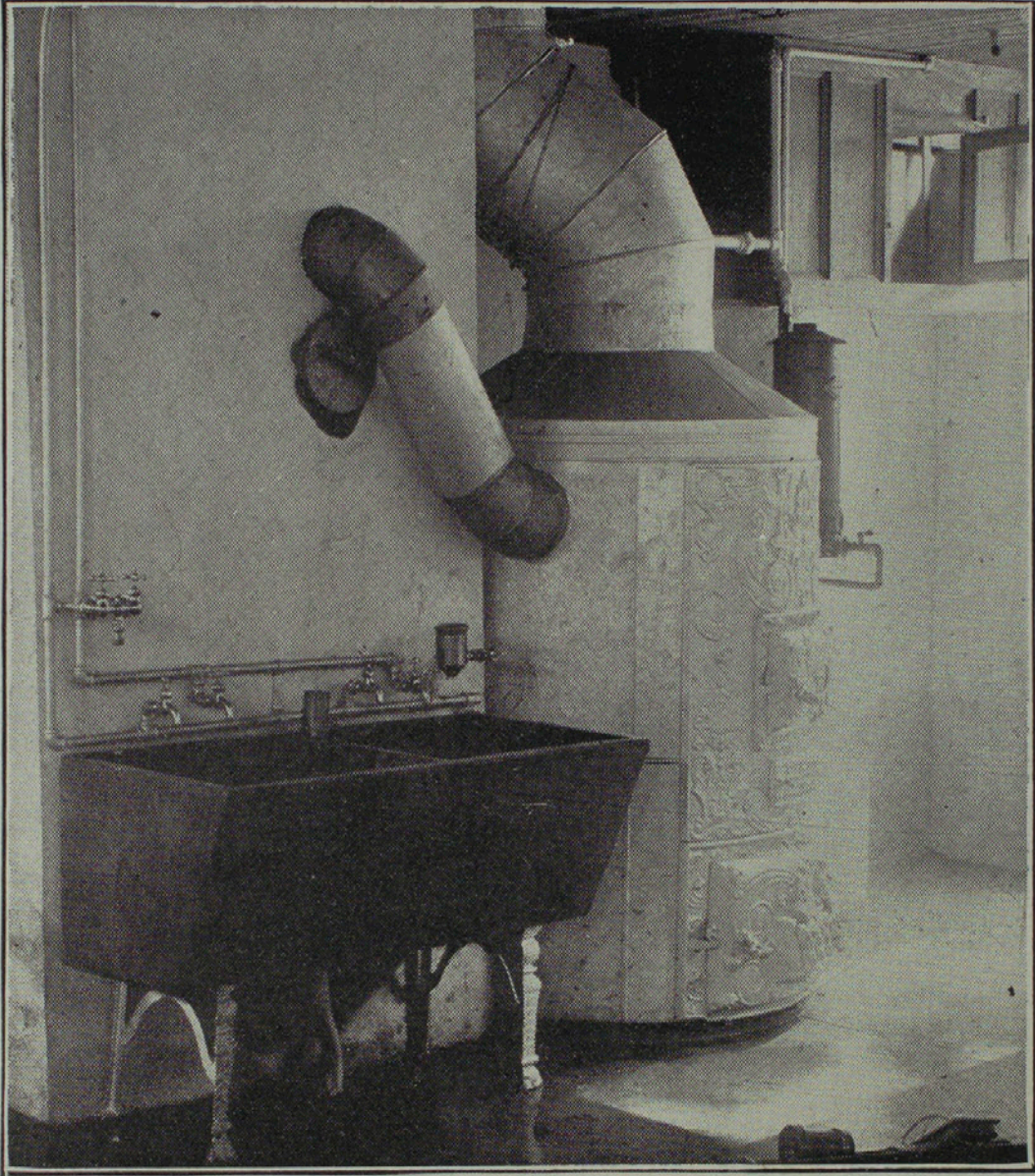
PARTS OF LAUNDRY AND FURNACE ROOMS, NOT YET SEPARATED BY PARTITION.
