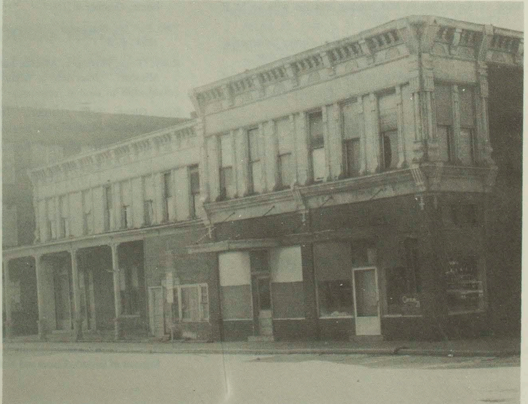
The Dockery Hotel in 1987 is showing its years of wear.
