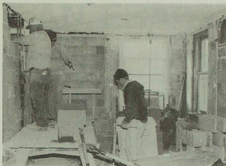
During the renovation men worked on installing new cement walls and a new plumbing system.
