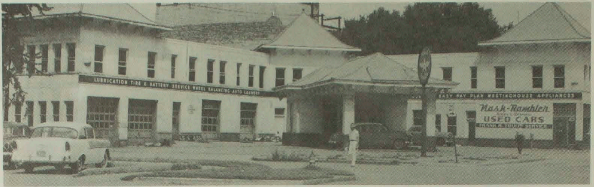
The present location of the Bank of Kirksville was the Truitt Garage on the corner of Franklin and Jefferson. This picture was taken August 14, 1958.
