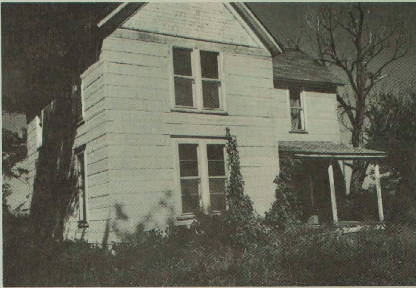
The north side of the old Schmoyer home place. It was built after the Civil War with materials from the bullet-proof house.
