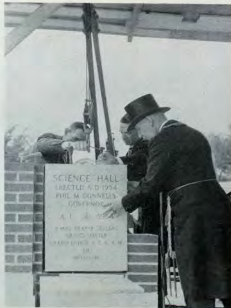
The Laying of the Cornerstone of Science Hall, J. MacBrayer Sellers, M. W. Grand Master, Grand Lodge, A. F. & A. M. of Missouri, officiating.
