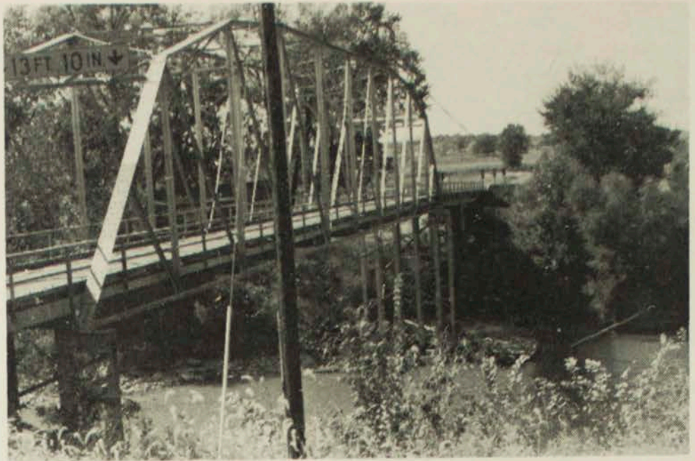
It took the people of Yarrow eight years to collect enough money to build the present Yarrow Bridge.
