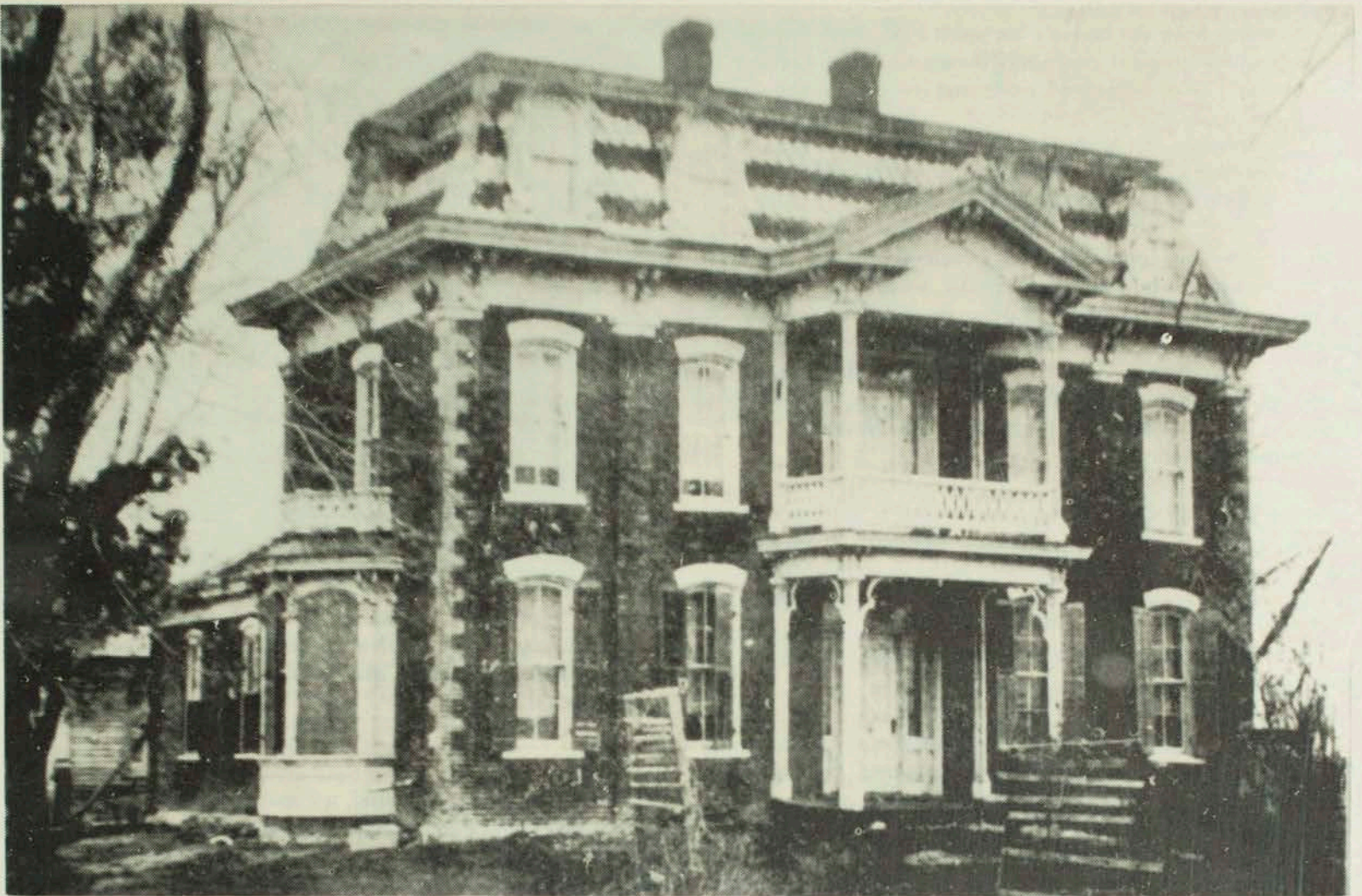
The huge, three-story brick Kellogg home was set back from the road, almost hidden by large trees. It stood on the land which is now the swim-
