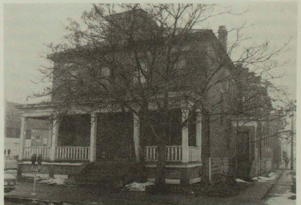
The Adair County Jail, which served Adair County for 68 years, was vacant for nearly two years before it was torn down in 1975 to make way for a new jail.
