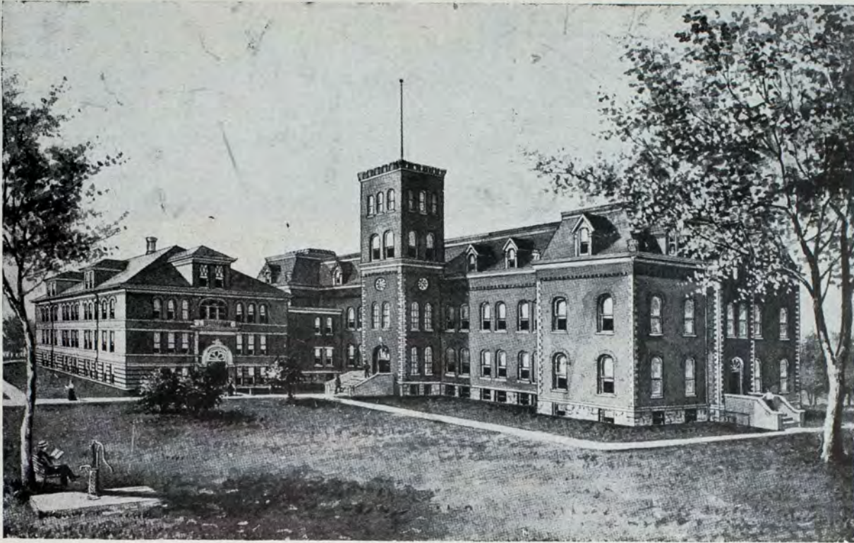
The library wing shown above was authorized by the Legislature in 1901. These two buildings were destroyed by fire in 1924.
