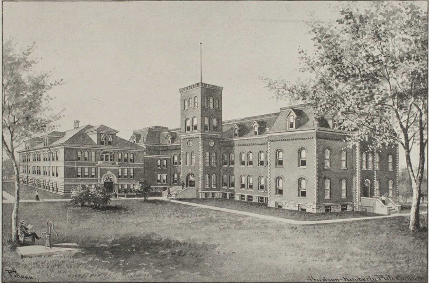
PRESENT BUILDING. ADDITION AT LEFT COMPLETED DECEMBER 25, 1901.
